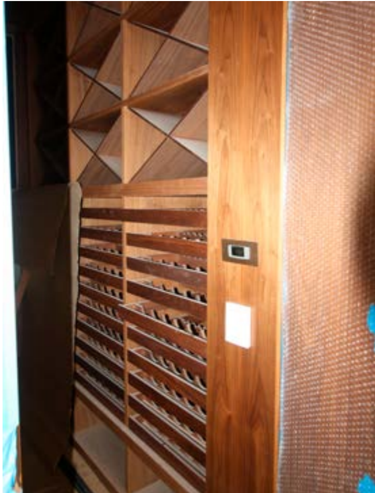
Construction details of the bottle holders, with high-capacity Blum hinges and details of the laser-perforated brass grid during assembly at the customer's villa.
